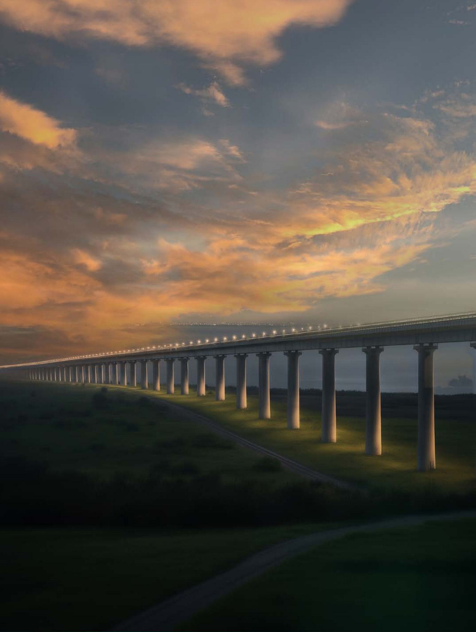
Nairobi Railway Bridge, Kenya
