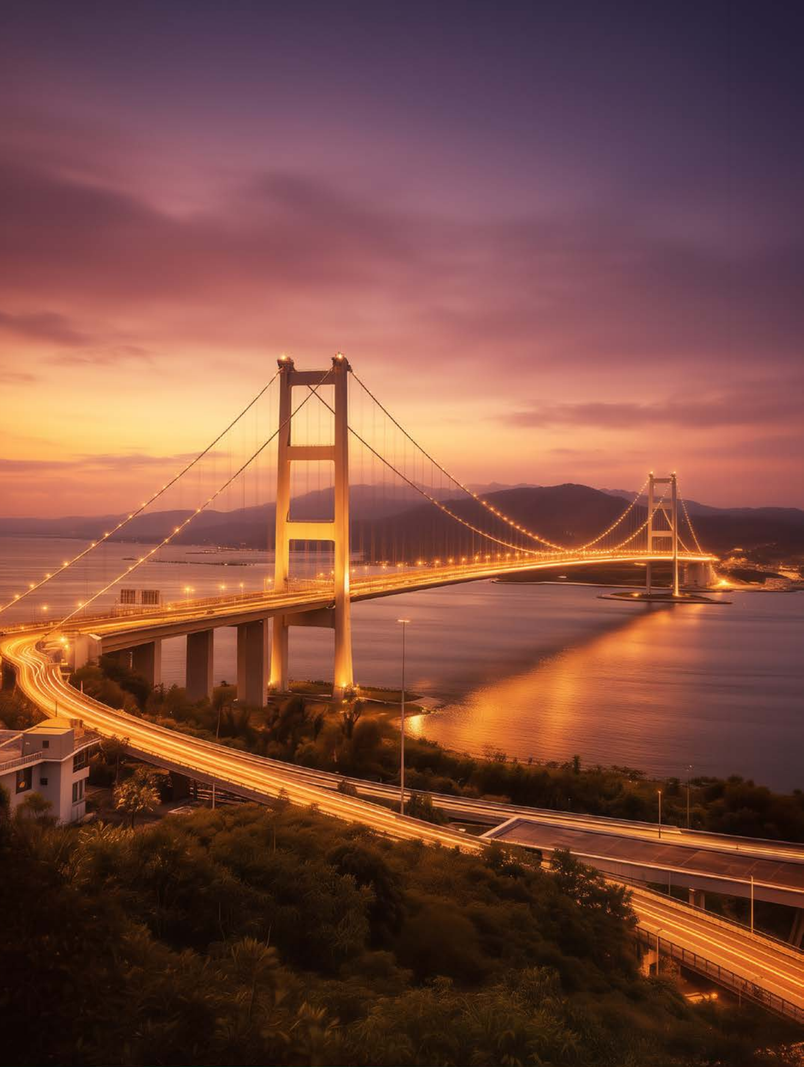
Tsing Ma Bridge, Hong Kong
